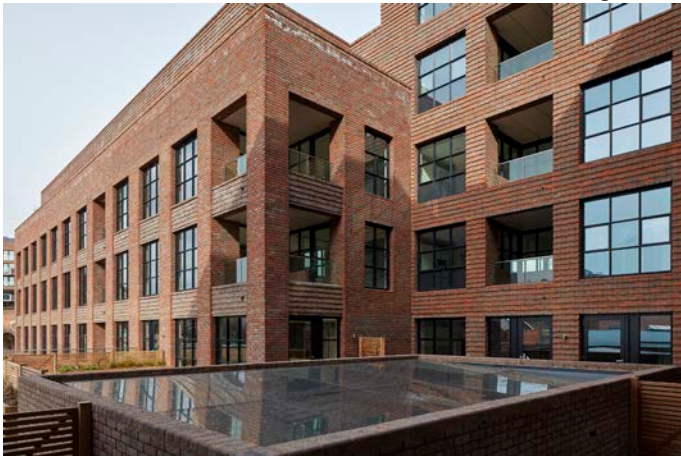
Brick mix and detailing variations are combined to enhance the materials palette
