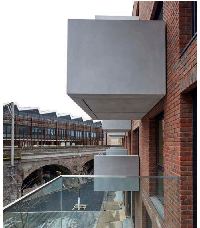
Staggered balconies face onto an open air market area at the centre of the site
