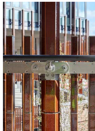
Horizontal bracing, handrail and joints
