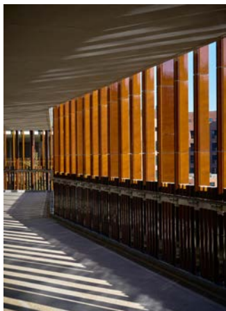
Internal view of terracotta
