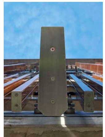
Steel caps at base
