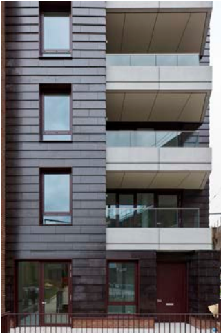
Hawley rd - north Terracotta, brick and GRC
