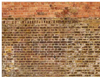
① Existing brickwork
