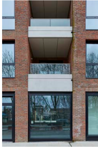
Castlehaven rd - west GRC with brick detailing
