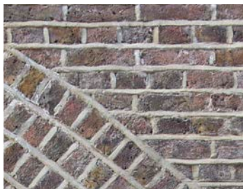
① Existing brickwork
